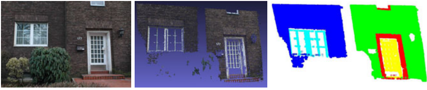
Fig. 3. Left: One of three images taken for a building facade scene. Middle: A snap-shot image of corresponding 3D point cloud generated by PMVS. Right: The five dominant planes automatically extracted from the point cloud.
