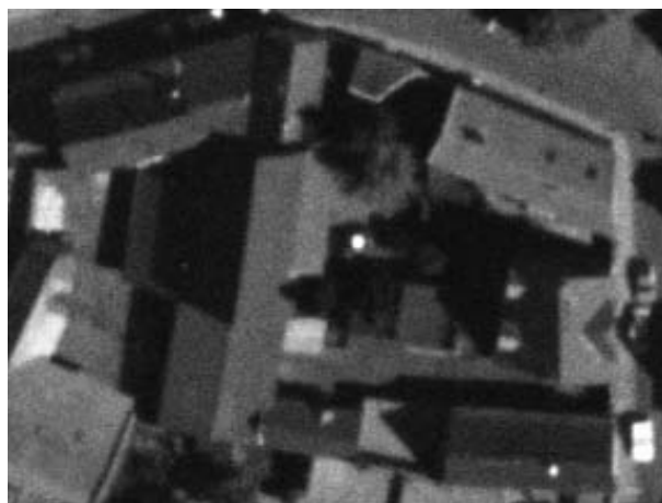
Figure 1: shows a section of an aerial image with some buildings, ©DeTeMobil GmbH, Bonn, 1998
