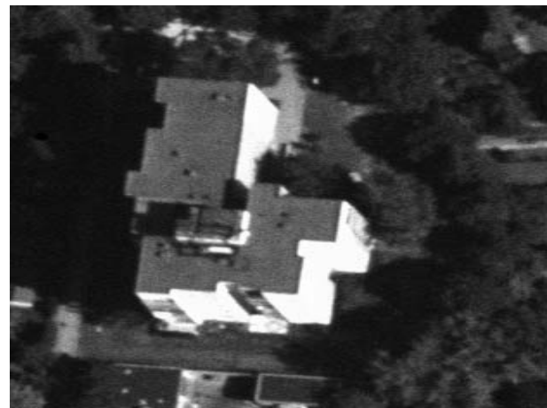
Figure 7: shows the original complex building ©DeTeMobil GmbH, Bonn, 1998
