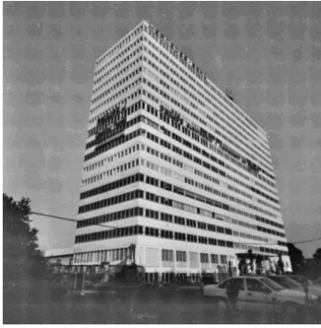
Figure 5: shows the image of a high building.
